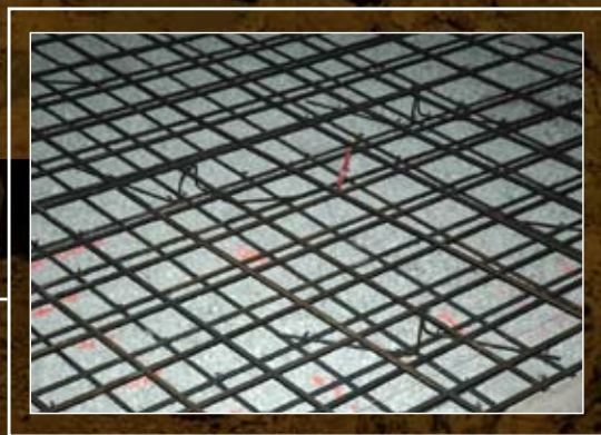
Rebar mat in concrete slab
